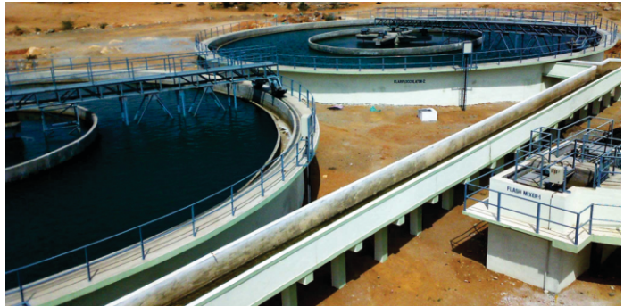
Sewage Treatment Plant (Only Plumbing)
